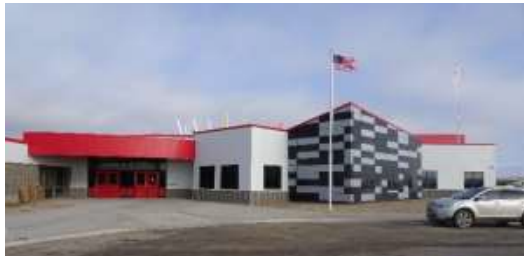
Wolf Creek Elementary School main entry
