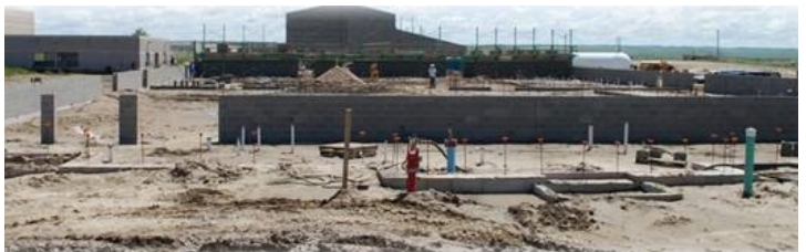
Early construction at Batesland School
